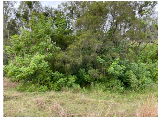
Photo 5.6. Weed proliferation in drainage line
